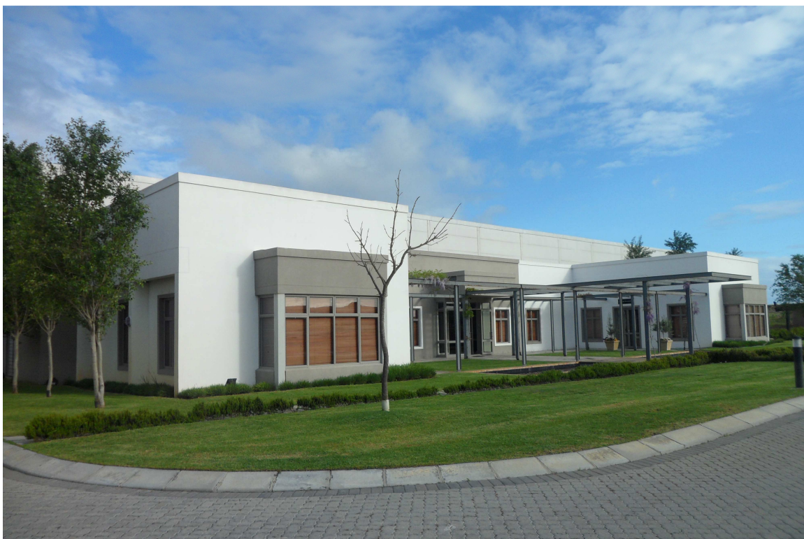
Picture 2: Labelling and wine storage facility of Compagniesdrift
