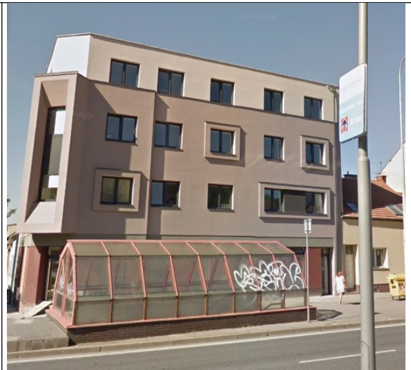
Figure 15 Refurbished and Extended Multifunctional Building on Mikšičkova Street [52]
