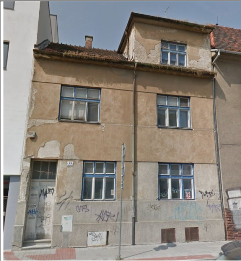
Figure 12 Apartment Building on Gajdošova Street before Refurbishment and Extension [52]
