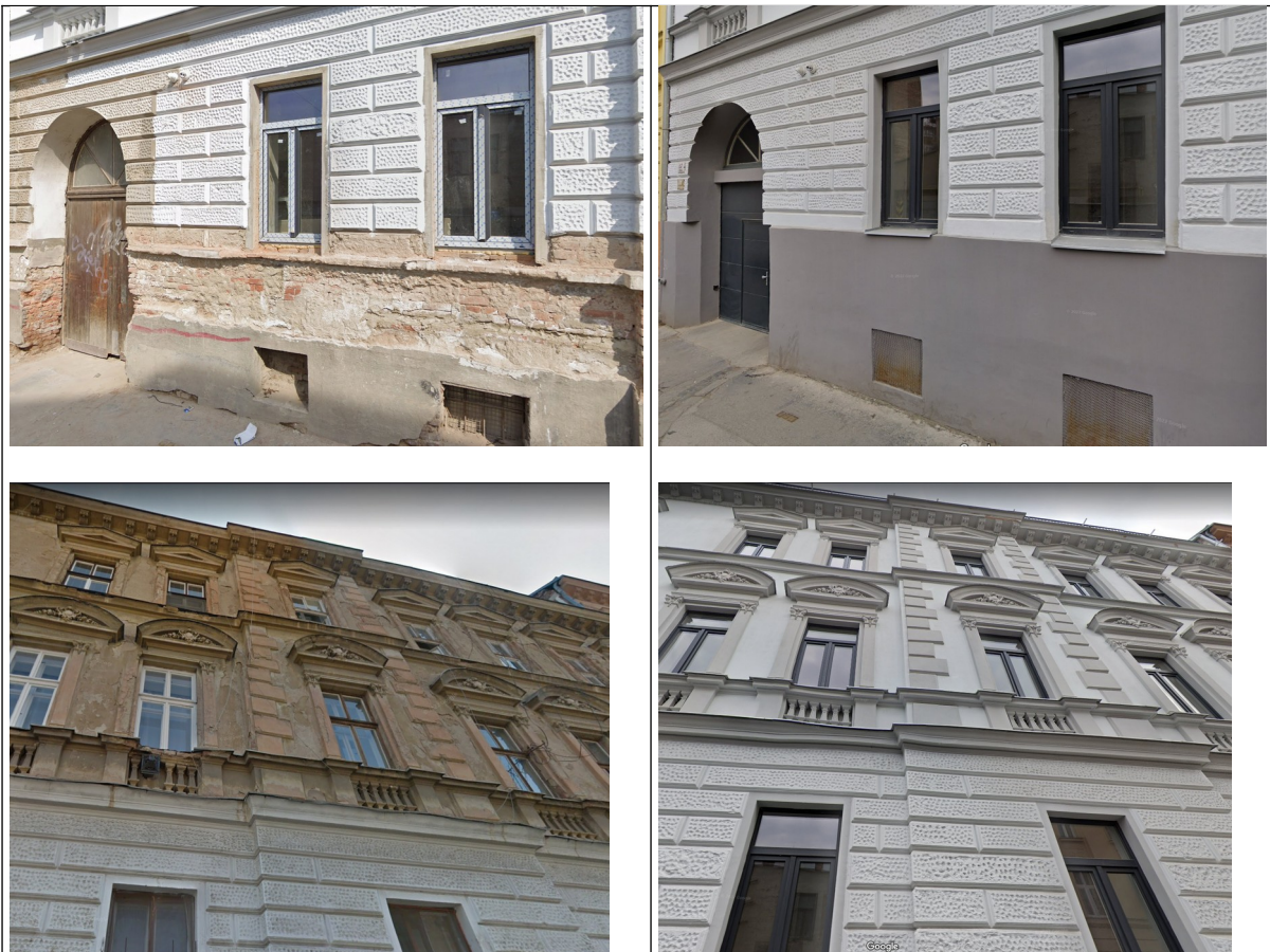
Figure 10 Apartment Building on Vlhká Street- before Refurbishment [52]
