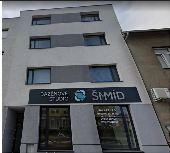
Figure 13 Apartment Building on Gajdošova Street after Refurbishment and Extension in 2018 [52]
