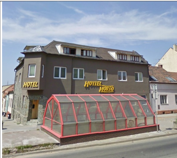
Figure 14 Former Hotel on Mikšičkova Street [52]
