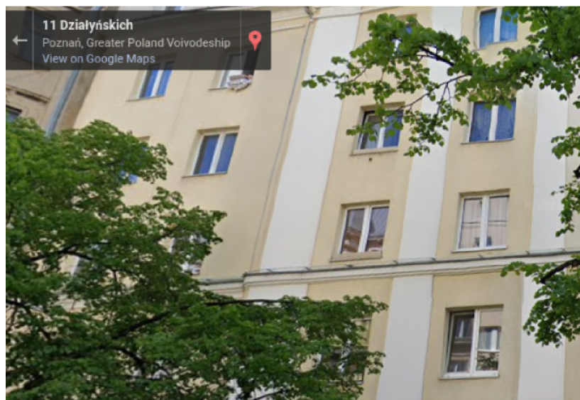
Figure 7.6: The same building found on the street that is mentioned in a Polish advertisement
