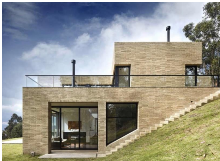
Figure 40: A Building located in high slope area (Laharchitect, 2020)
