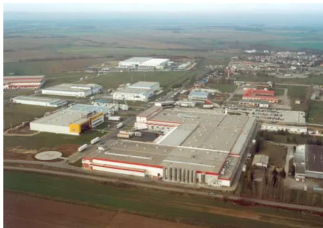
The Flextronics facilities in Sárvár, 2006
