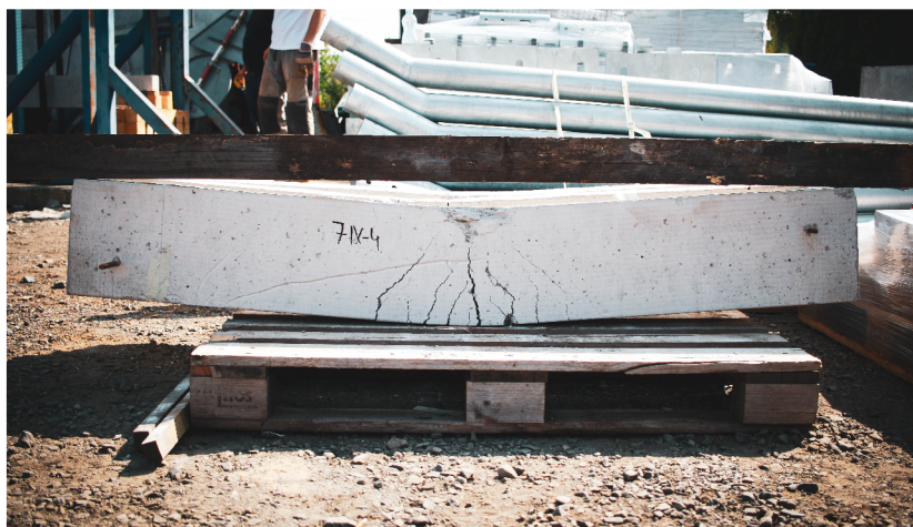
Fig. 8.2. Damaged specimen 7IX-4 after the impact.
