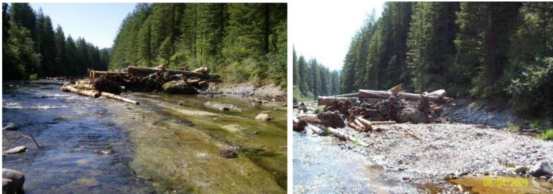
Image 7: Wooden structure forming gravel bed (Cramer 2012).
