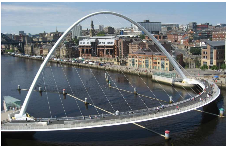
Obr. 35 – Gateshead Millennium Bridge, Newcastle upon Tyne, Anglie, UK
