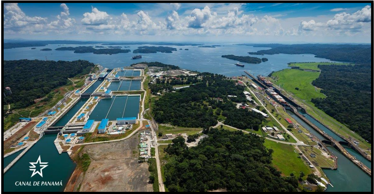
Figure 2: Expansion of the Panama Canal.
