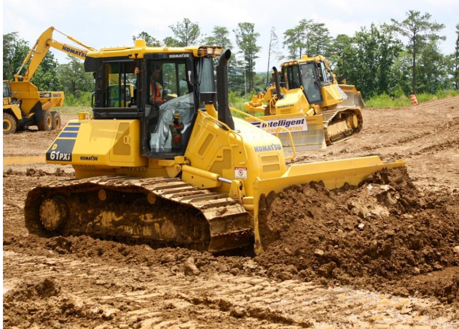
Obr. 3 Dozer Komatsu D61i
