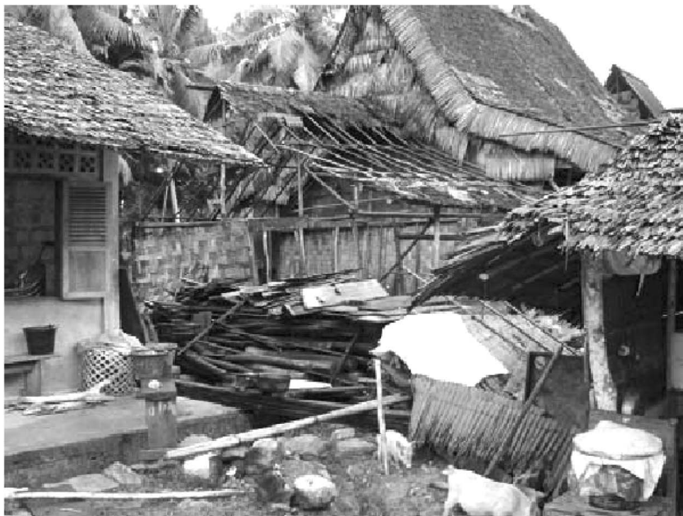
Zdroj: Boen, T. (2006), Structural Damage in the March 2005 Nias-Simeulue Earthquake
