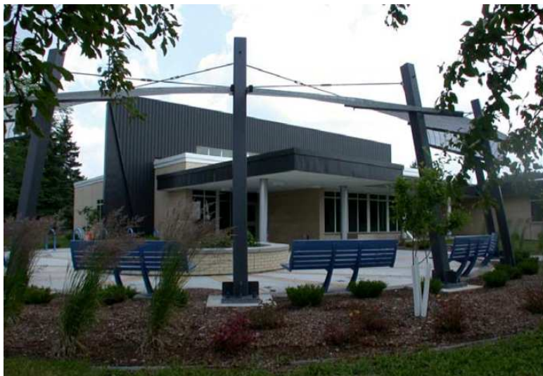
Obr. 5.12 Hibbing Courthouse Annex, St. Louis County (USA); [9]
