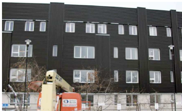
Obr. 5.5 Flin Flon General Hospital s instalací SolarWall®, Flin Flon Manitoba (Kanada); [9]
