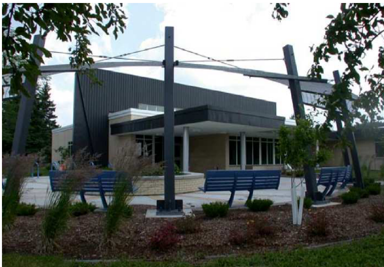
Obr. 5.12 Hibbing Courthouse Annex, St. Louis County (USA); [9]
