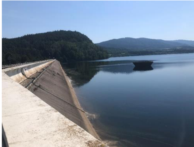
Figure 7. The dam of the water reservoir Nýrsko (author's photo)
