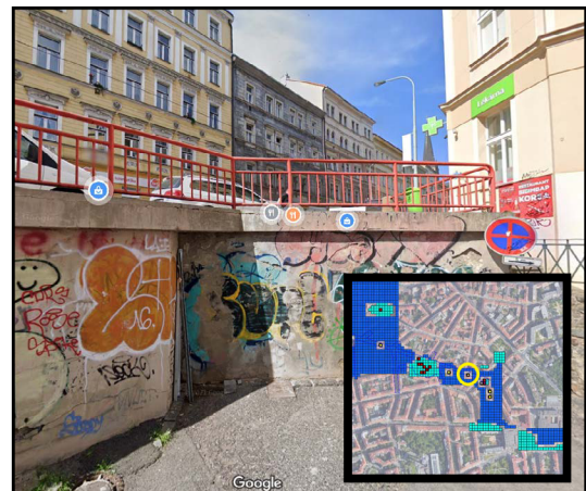
(fig-30) safety concern hot-spot near the Lipanska street intersection, as indicated in the model. [Google street view 2023]
