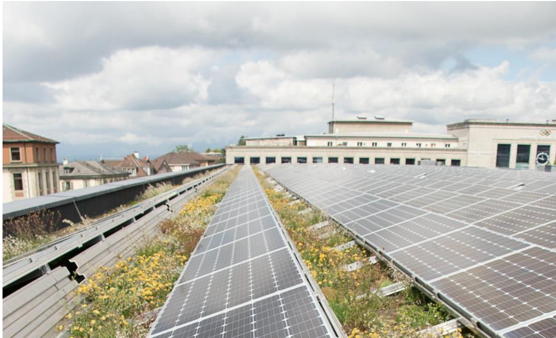
Figure 10: Biosolar green roof of the Palais Beaulieu in Lausanne, Switzerland (Catalano and Baumann 2017)
