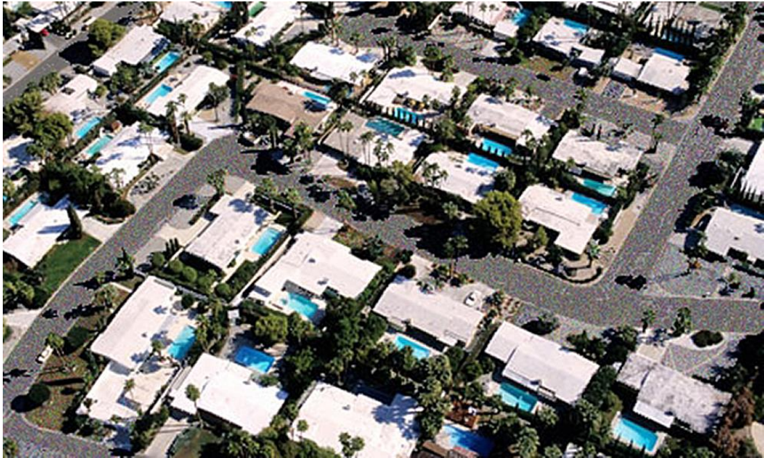
Figure 8: In California, flat-roofed houses are now required to have white roofs (LA Weekly 2009).
