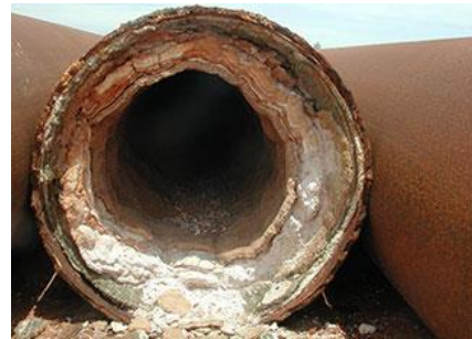
Figure 8. Fouling on heat exchanger.
