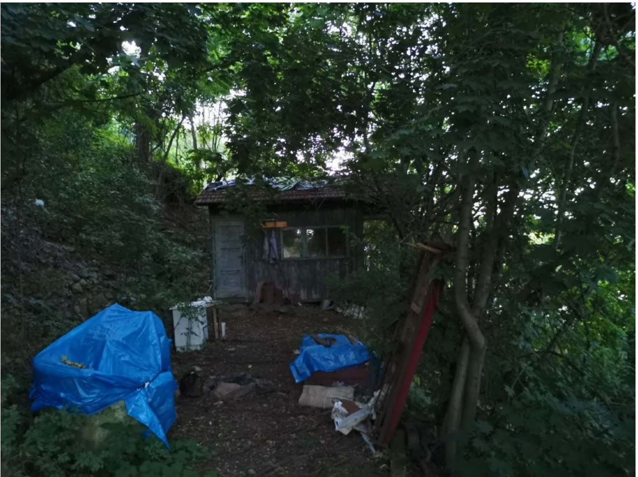
Figure 3: Current state of exterior and of surroundings of the ssesi.space.
