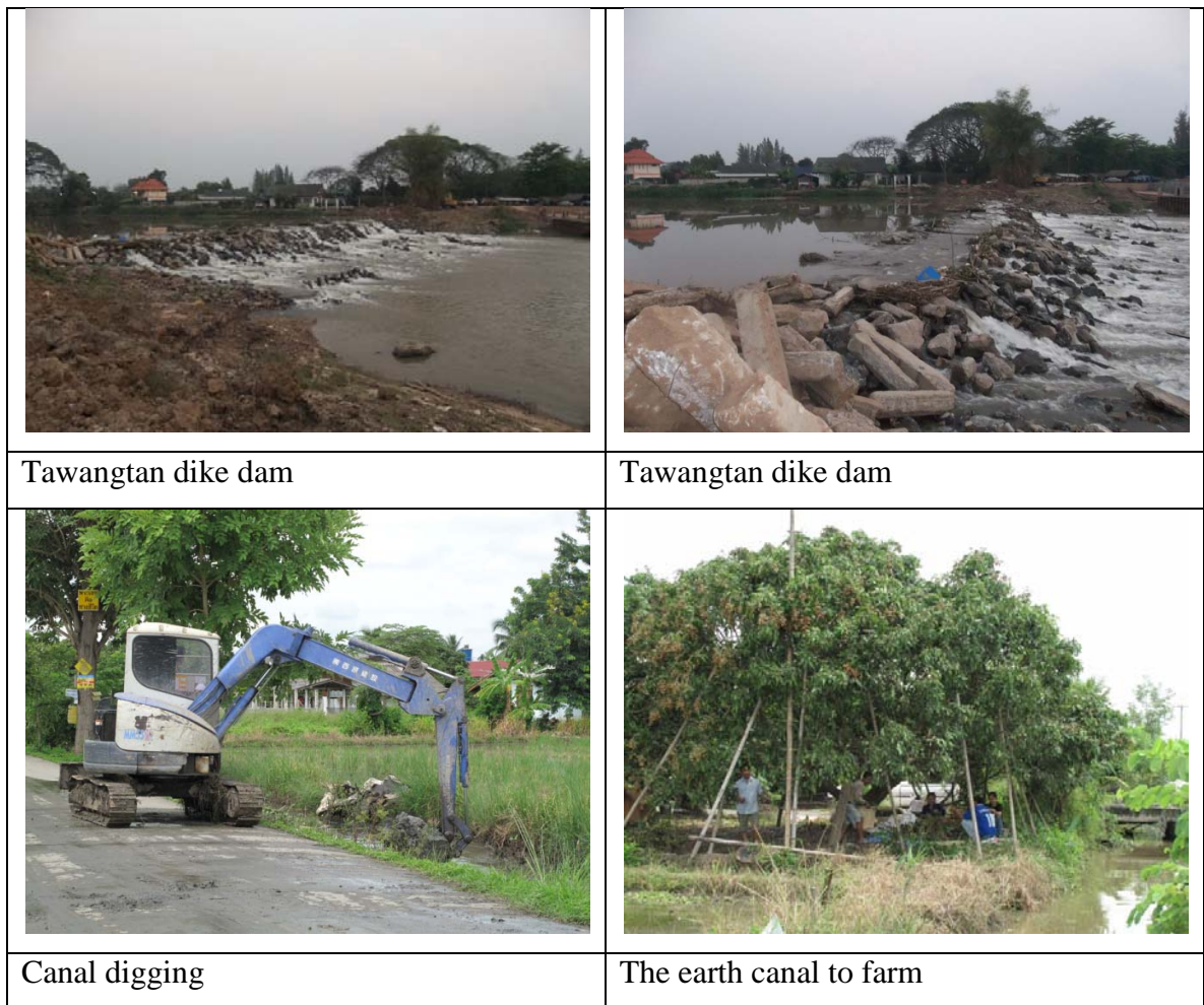
Figure 11 Water resource in dike dam is Tawangtan Muang Fai
