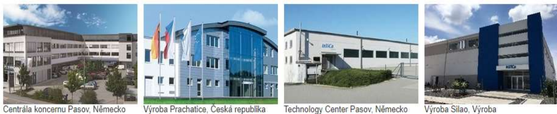
Obr. 2.2 InTiCa Systems AG / lokace.
