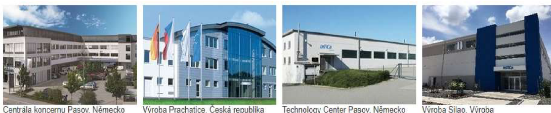
Obr. 2.2 InTiCa Systems AG / lokace.
