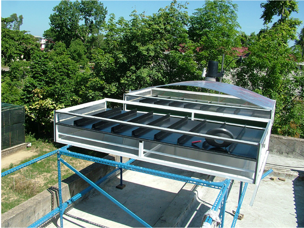
Construction of solar dryer.
