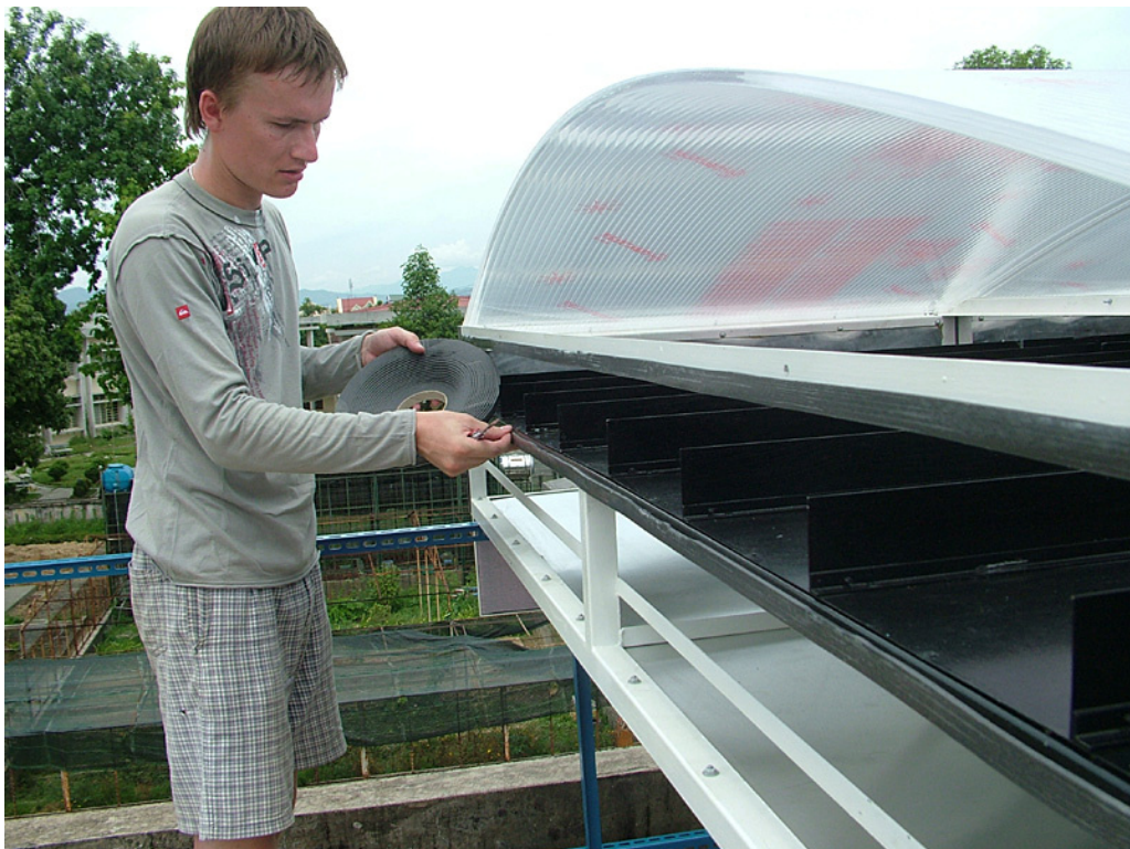
Placing the insulation tape between two segments of solar dryer.
