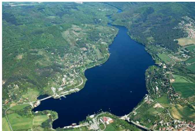
Picture n. 4: Brno dam
