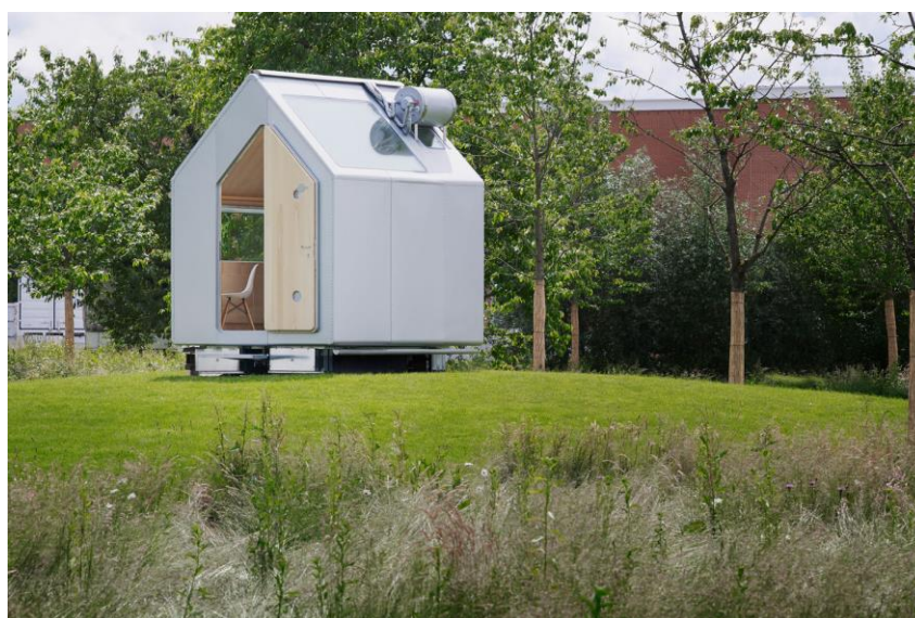
Obr. 28: Diogene House – exteriér
