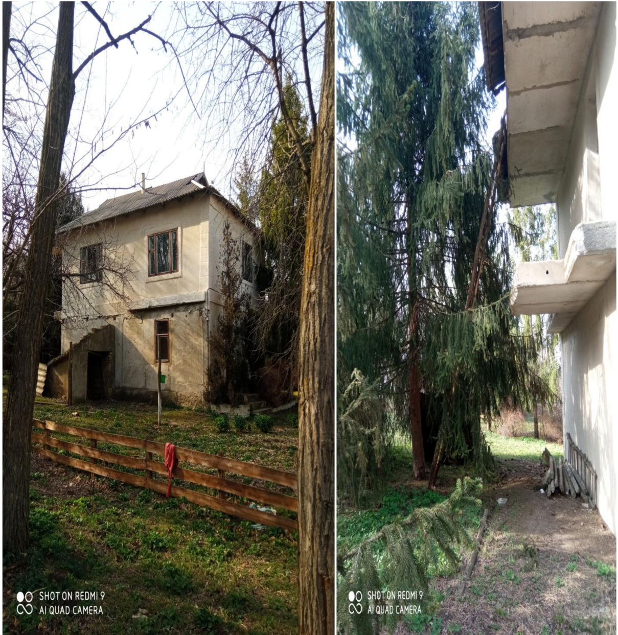
Photos 11 and 12. Forest range Nr.3 house and ladder to the attic
