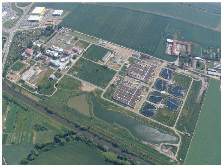
Obr. 7 ČOV Brno – Modřice [16]
