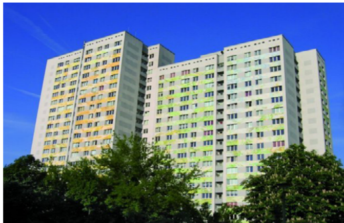
Figure 11: Block of flats in Włochy District
