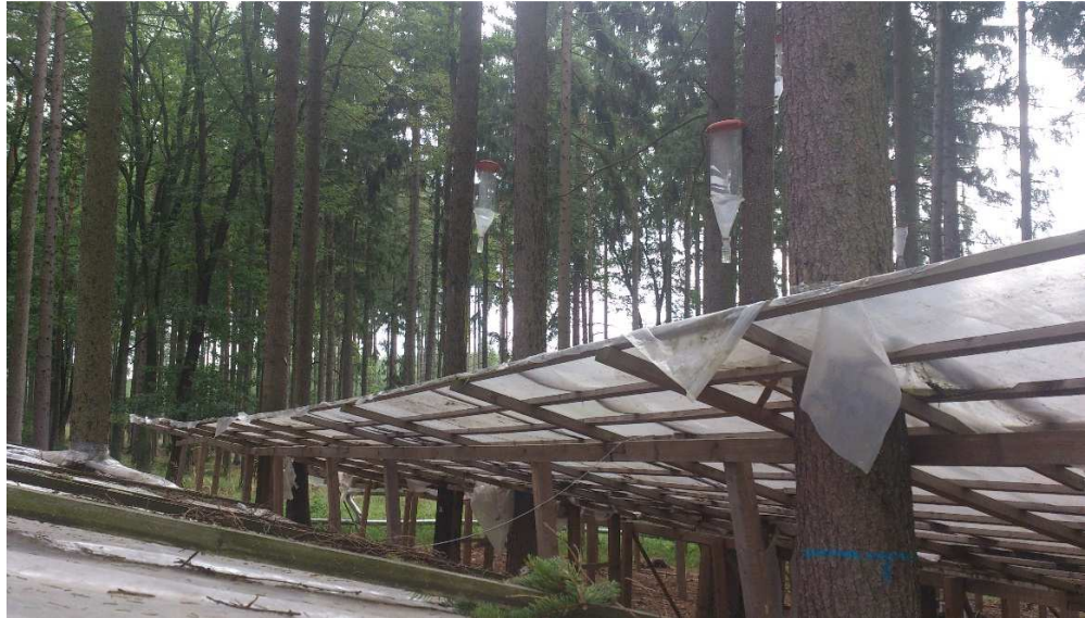
Photo 9 – Roof system in the experimental plot. (Mladenović Strahinja, 2013)
