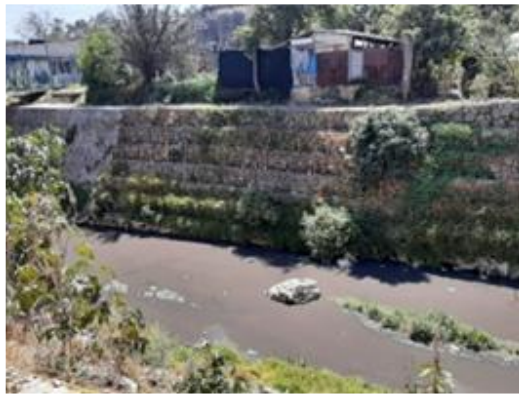
Picture 2: Gabion wall at zone “25 Zona Militar” in Puebla City. Source: Self-made picture
