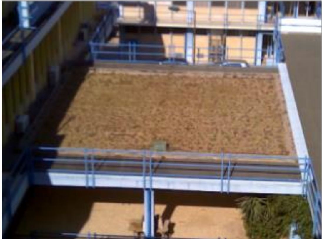
Figure 32. High-angle view from the rooftop of the faculty building Source: Author
