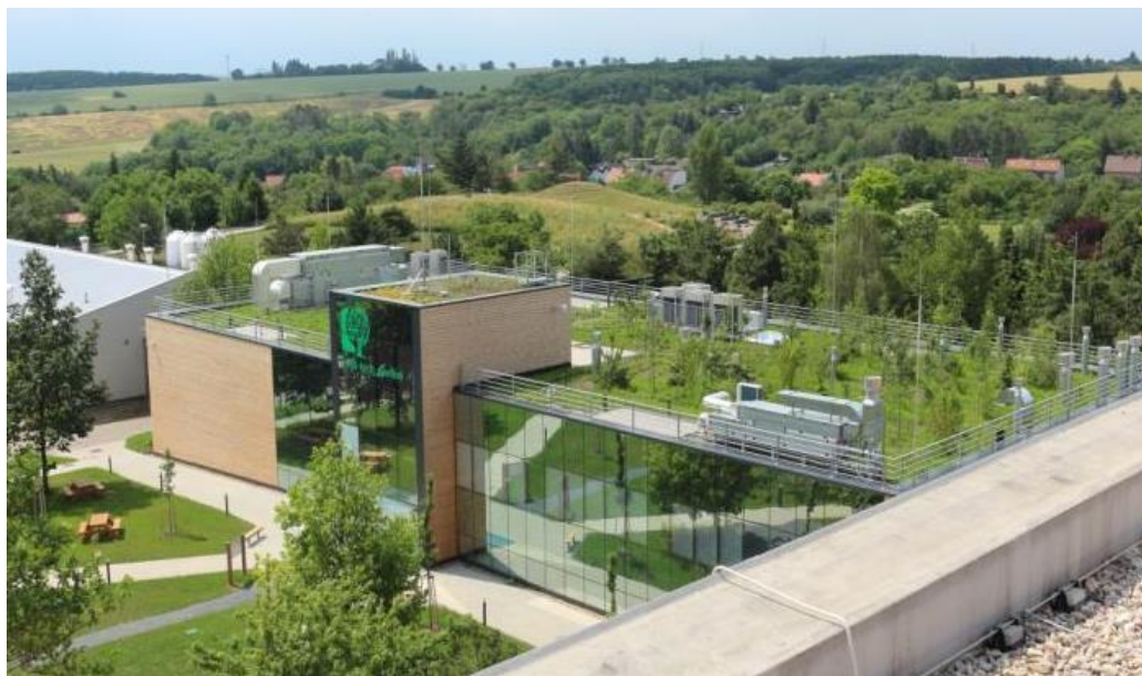
Figure 3. Green roofs of the High-tech Educational Pavilion of the Faculty of Forestry and Wood Sciences CULS in Prague
