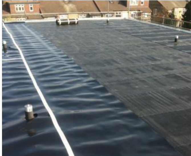
Figure 7. Photo of root barrier layer and water-proof layer
