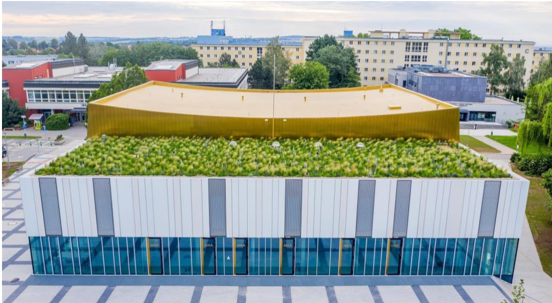
Figure 22. Aula green roof
