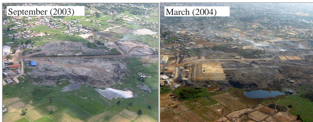
Figure 10. SMCD before and after pilot project. Source: (Kokusai Kogyo, 2005)
