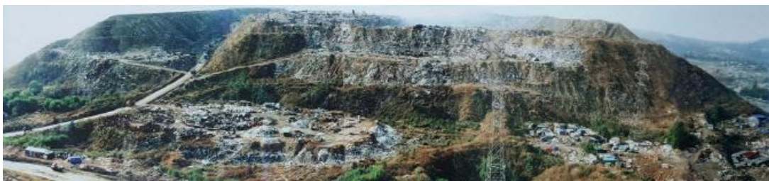
Figure 15. Najido dumpsite before redevelopment. Source: Seoul Metropolitan Government
