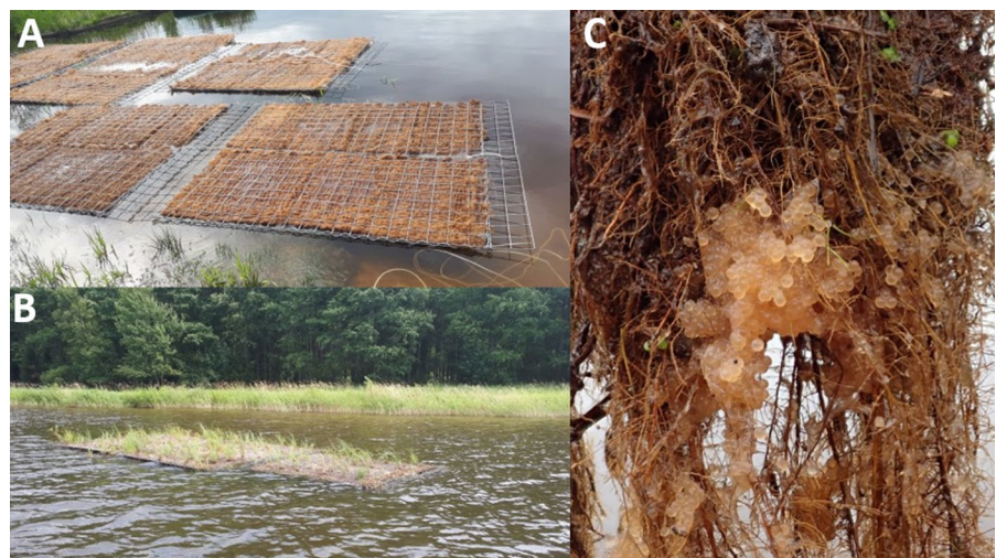
Fig. 3 Details of floating islands construction. A Freshly made elementary units of AFI before planting the plants. B Complete AFI-M2 in summer during the experiments. C Roots of plants hanging down from the AFI in April 2019 with the eggs of roach
