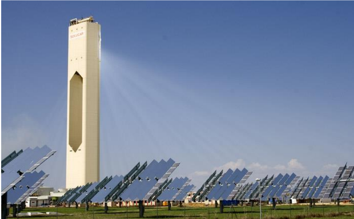
Fig. 3-7 Concentrating solar power plant Planta Solar 10 (11 MWp) in Seville, Spain 14
