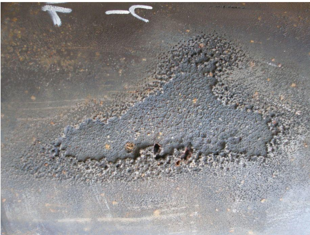
Corrosion – areal corrosion – Diesel motor cylinder liner
