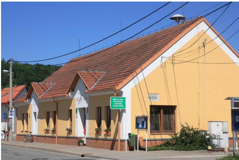
Figure 9 The municipal office of the community Ochoz u Brna
