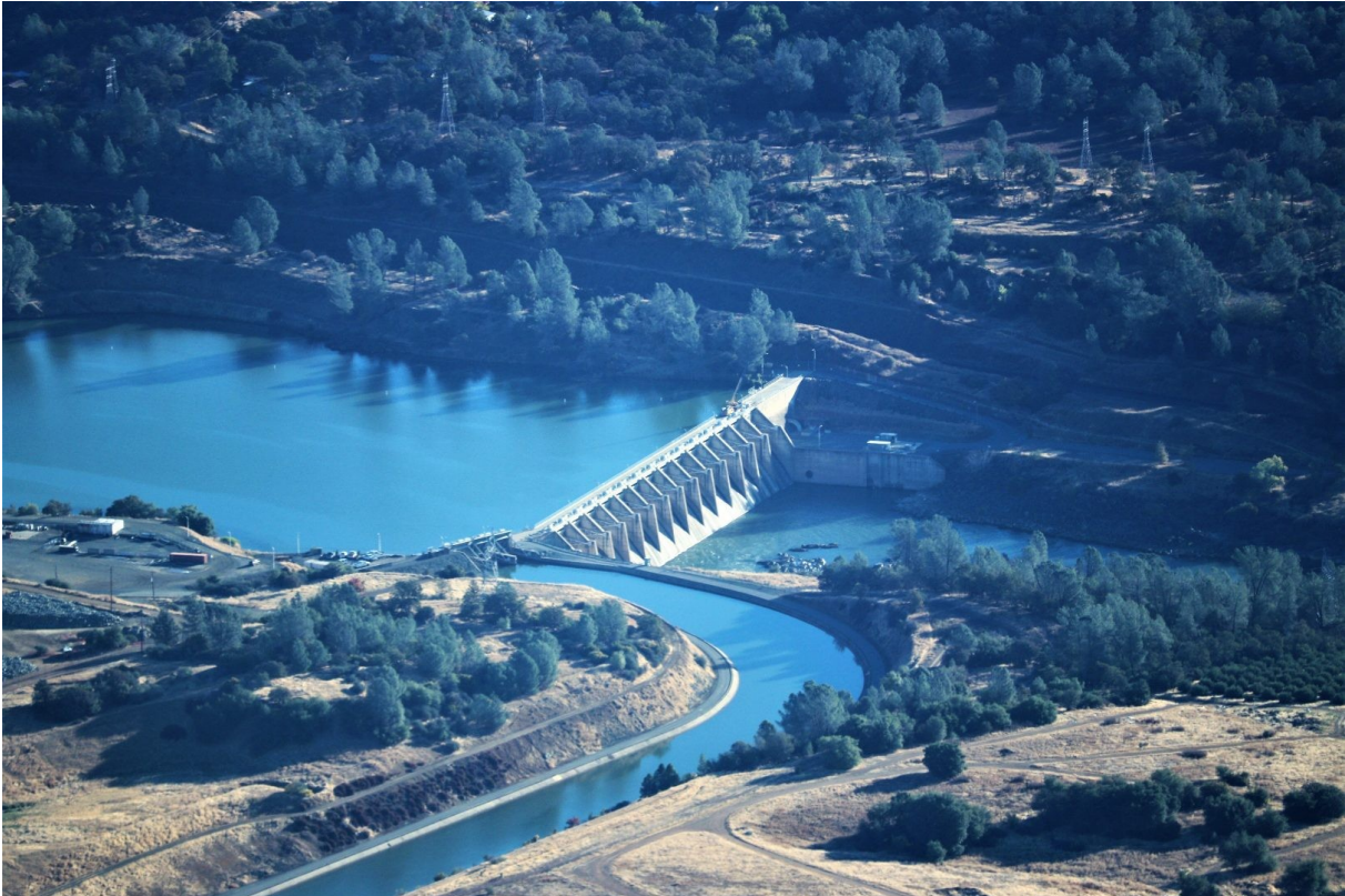
Obrázek 9. Thermalito Diversion Dam, Forebay and Thermalito Power Canal.
