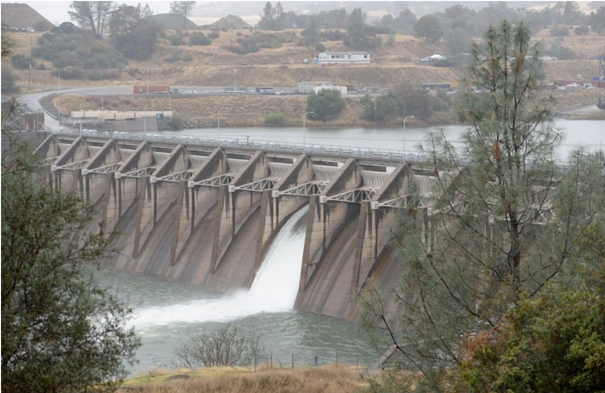
Obrázek 8. Thermalito Diversion Dam. Zdroj: https://mng-chico.smugmug.com/Oroville-Week-of-11-20-2017/i-dFMPrPd
