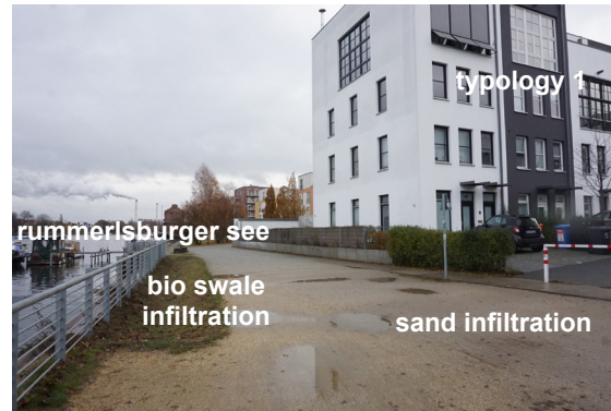
Image 14: The area between typology 1 and the Rummelsburger See consists of sand and gravel paving and a vegetative retention strip running parallel to the water's edge to reduce the amount of point source pollution from surface water runoff.
