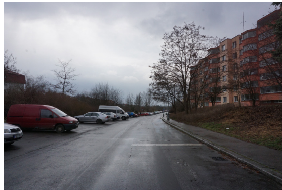
Image 44: In the case of Černý Most, the roads, sidewalks and secondary paths are all made of asphalt material. For this reason, all asphalt areas are calculated as 'roads', with a runoff coefficient of 1.0, in the peak discharge calculation (Photo by author).
