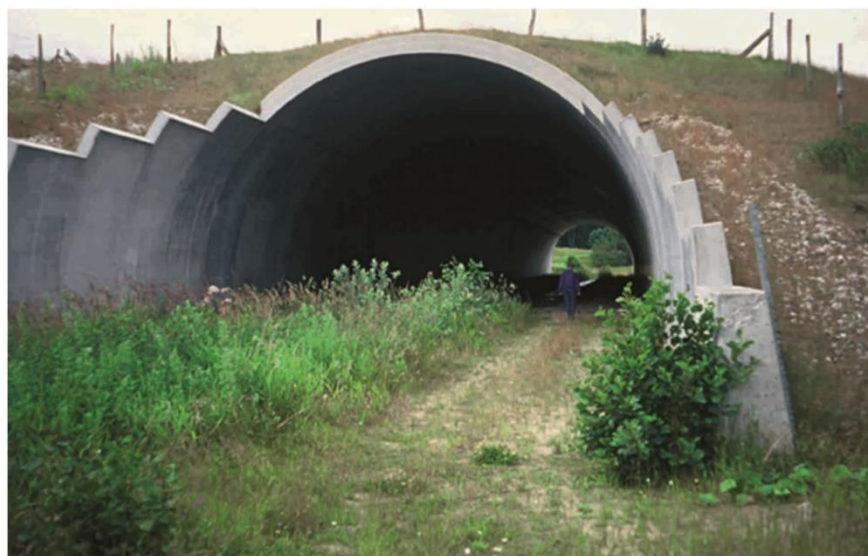
Fig. no. 3: Underpass in Denmark ( www.handbookwildlifetraffic.info )
