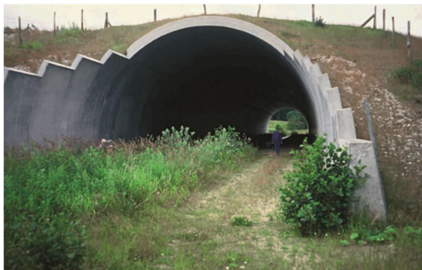
Fig. no. 3: Underpass in Denmark ( www.handbookwildlifetraffic.info )
