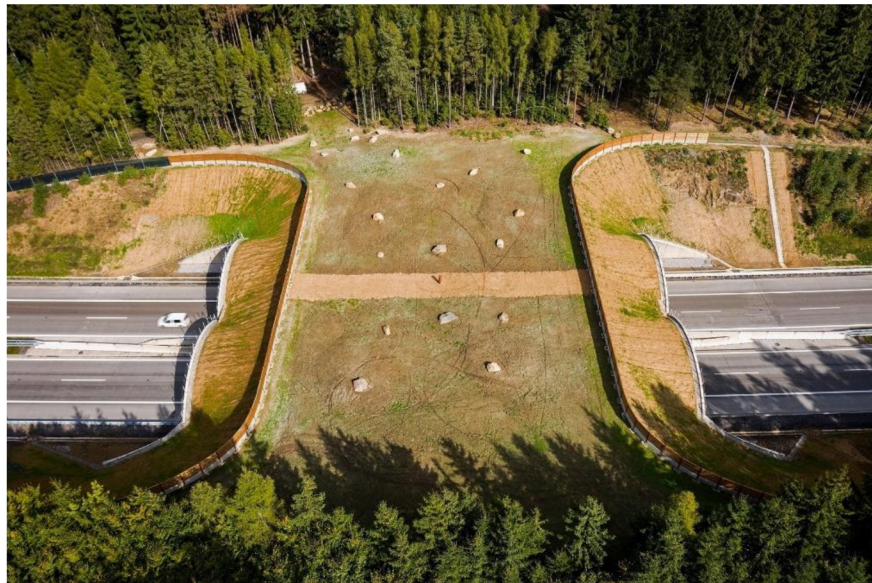
Fig. no. 2: Overpass on the D1 motorway, Czech Republic ( www.skanska.cz )
