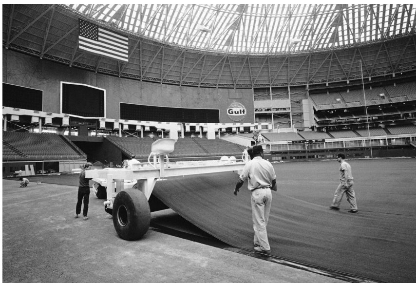
Obr. 1 Instalace povrchu Chemgrass v hale AstroDome [4]
