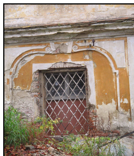
Obr.73 - portál vjezdu detail
