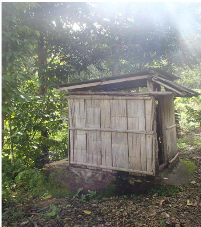
Figure II: Single-vault composting toilet with bamboo superstructure
