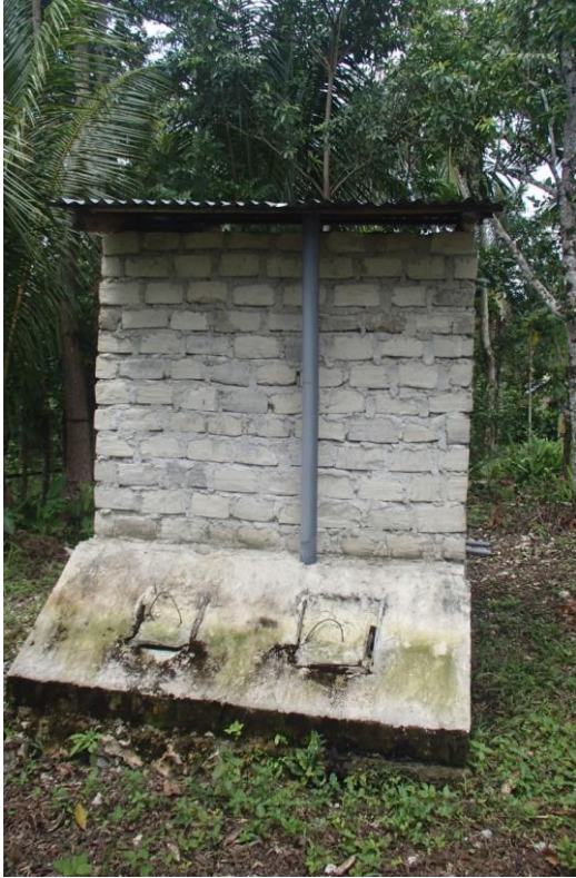
Figure III: Double-vault composting toilet with urine-separation with back side doors to access the compost.
