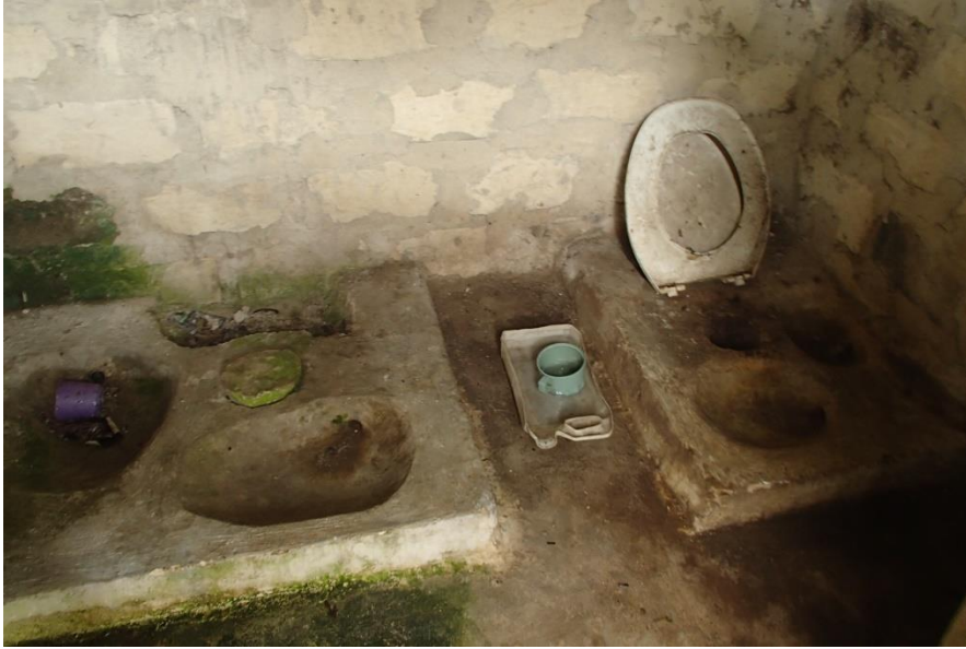
Figure V: Interior of double-vault composting toilet with three holes for separating urine, excreta and water used for anal-cleansing.
