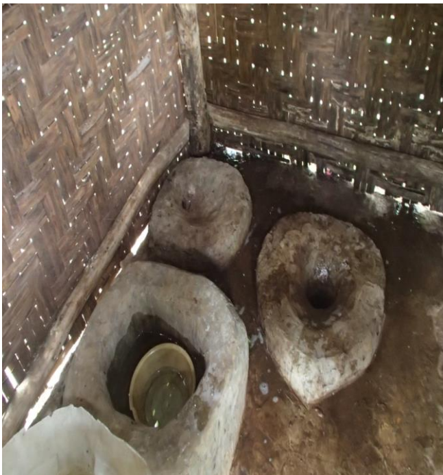
Figure IV: Interior of composting toilet with water collector and designated place for anal-cleansing and urine.
