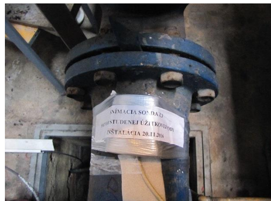
Picture 3.25. – Left: Temperature sensor at cooled natural healing water (green pipeline), right: Temperature sensor at cold service water (blue pipeline)
