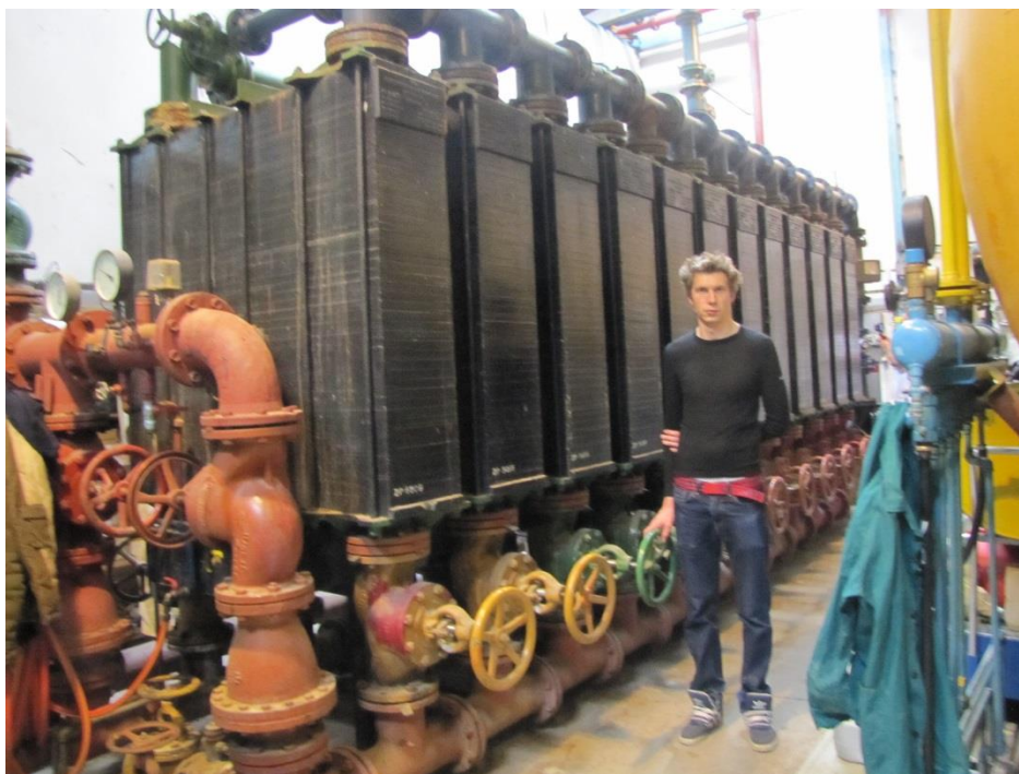
Picture 3.24. – Korobon block graphite heat exchanger
