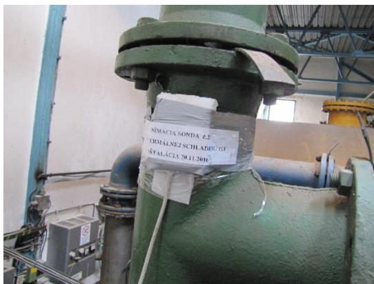
Picture 3.25. – Left: Temperature sensor at cooled natural healing water (green pipeline), right: Temperature sensor at cold service water (blue pipeline)
