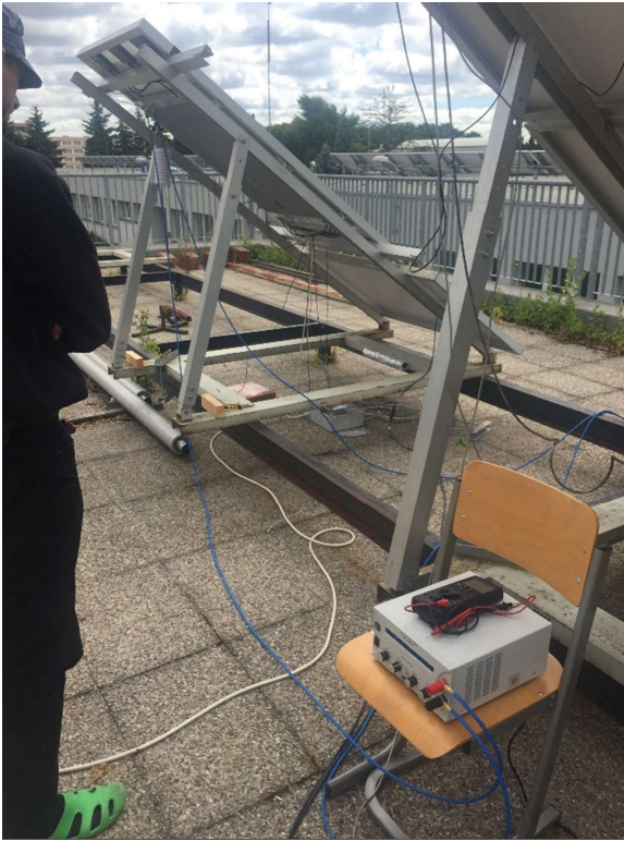
Figure 13. Measuring electrical characteristics of the PV-battery module prototype
