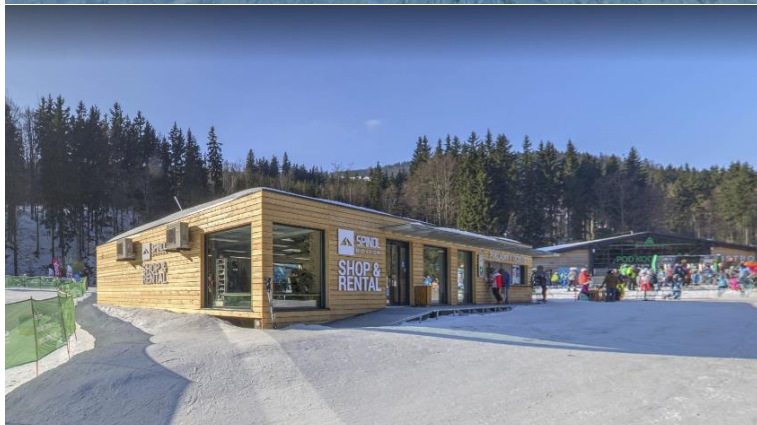
Obr. 18 Budova pokladny ( https://www.google.cz/maps/@50.7335319,15.6066972,3a,75y,16.85h,91.07t/data=!3m8!1e1!3m6!1sAF1QipPlo4xjoEcGpafixF6rJtZw9fTi6wyMslookwl8!2e10!3e11!6shttps:%2F%2Fih5.googleusercontent.com%2Fp%2FAF1QipPlo4xjoEcGpafixF6rJtZw9fTi6wyMslookwl8%3Dw203-h100-k-no-pi-0-ya107.48832-ro-0-fo100!7i9540!8i4770 )
