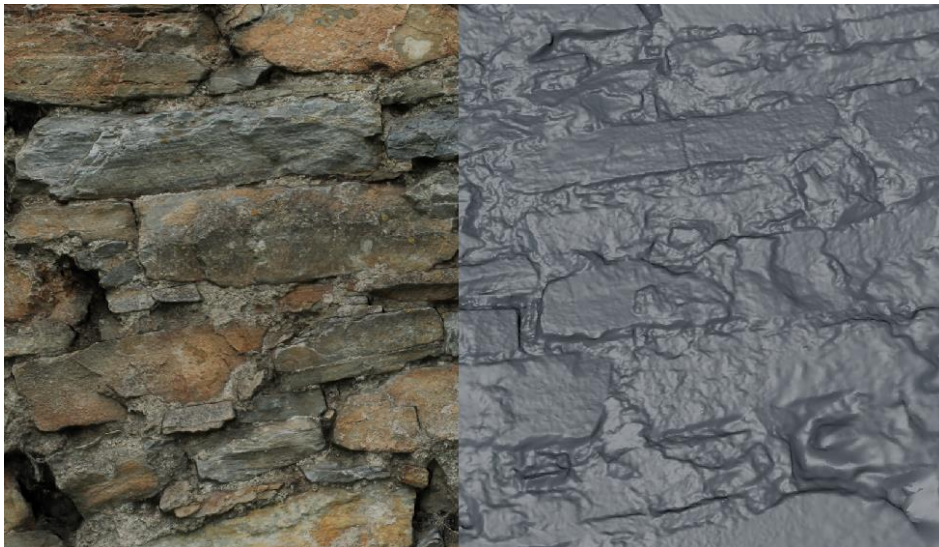
Obr. 24 – 3D sken s texturou a bez ní
