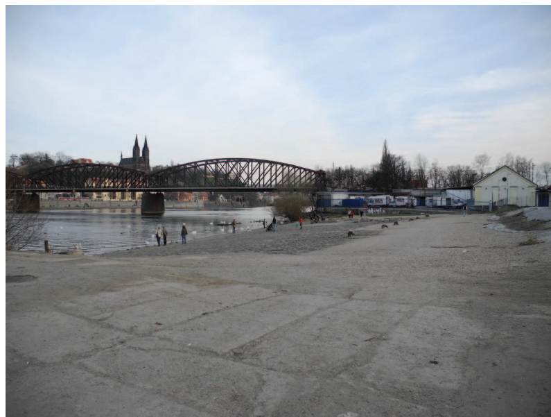
Figure 5.11: Current state photo of “Smíchov beach”
