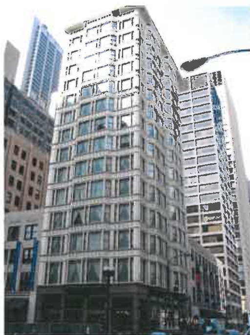
Obr. č. 31 – Daniel Hudson Burnham–John Welborn Root, Reliance Building, Chicago, USA, 1890–95.
