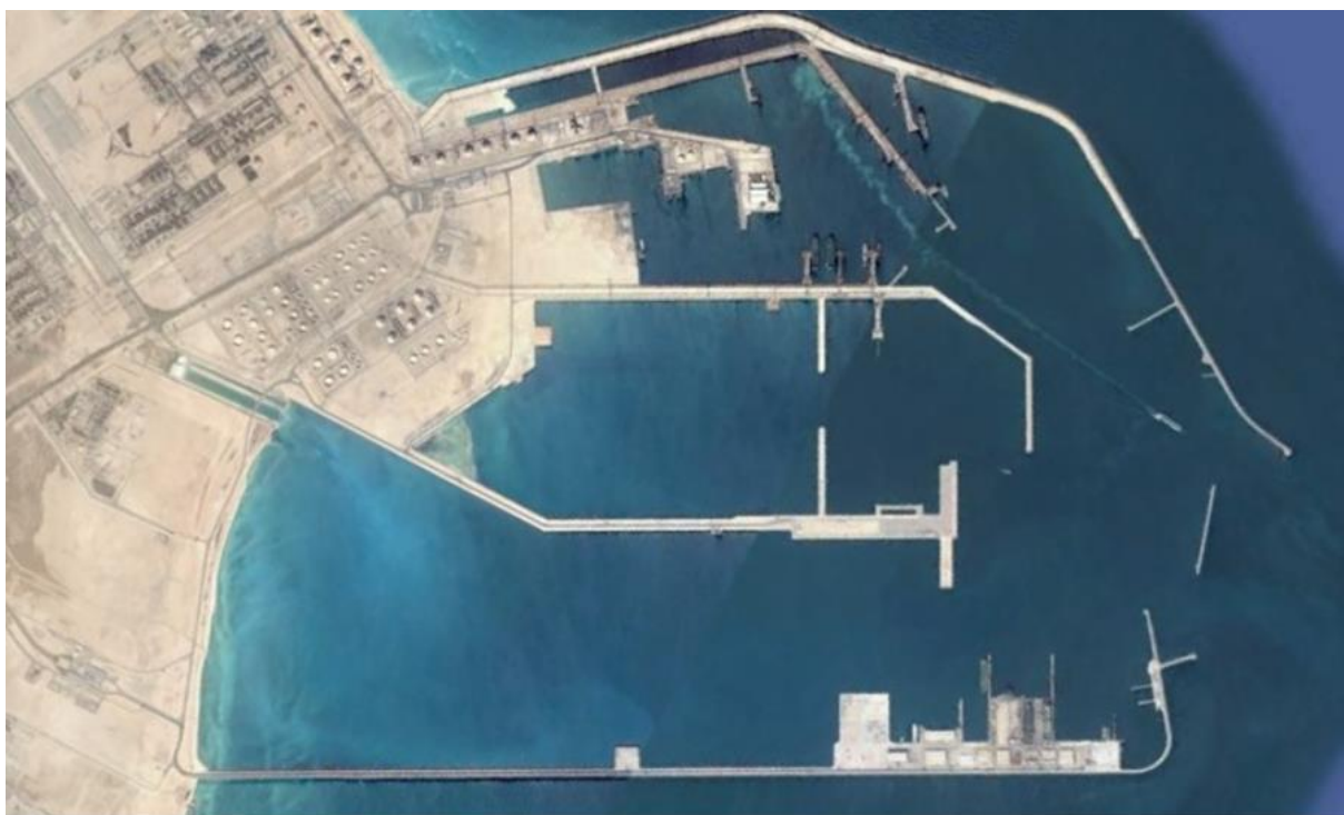
Figure 13: Arial View of Ras Laffan Port
