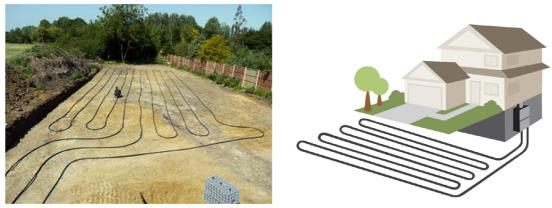
Picture 2.13. – Horizontal ground source heat pump [42],
