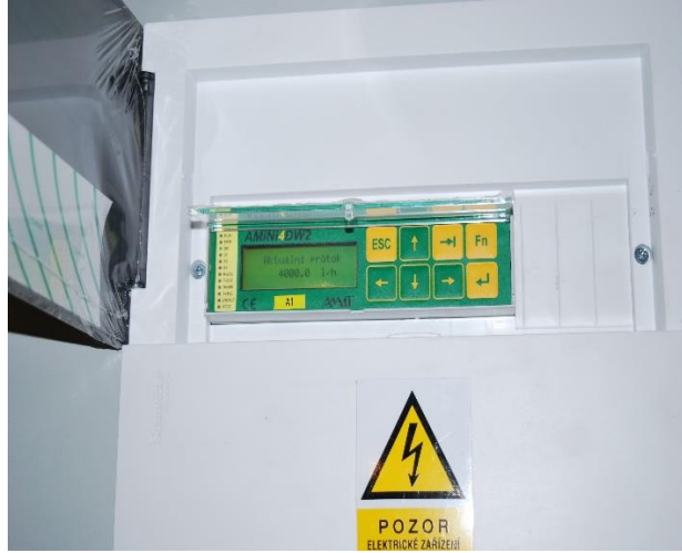
Figure 4.10 – Water meter G. GIOANOLA, IARC/25 R80, Class T90 with MaR recording system.
