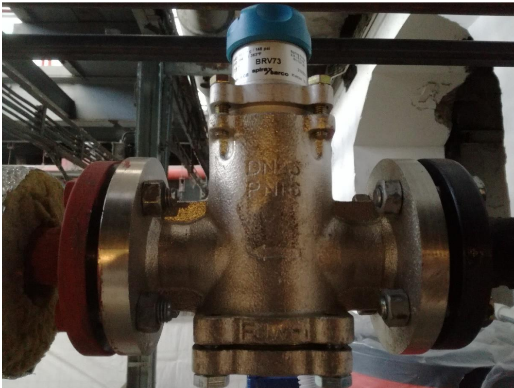
Figure 4.12 – Manual valve for pressure regulating by Spirax Sarco BRV73.
