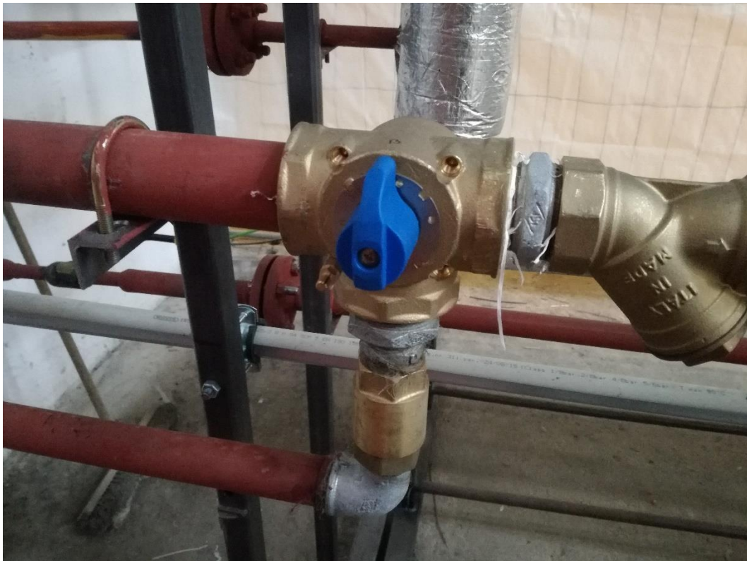
Figure 4.11 – Manual three-way valve.
